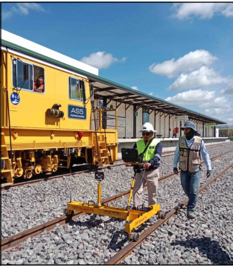
In the field with the Amberg GRP 1000 railway surveying system.
